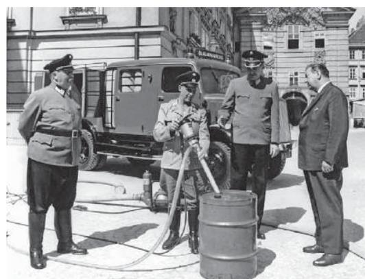
The world's first electric drum pump in operation.
